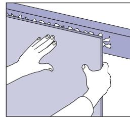
**6** Rub the back of each panel with coarse sandpaper in the areas that will make contact with the adhesive. Work with one sheet at a time, applying adhesive and installing. Position the panel carefully and press firmly to make contact with adhesive. Remove the panel until the adhesive becomes touch dry (approximately 5 to 10 minutes) and follow the adhesive manufacturer's instructions.
